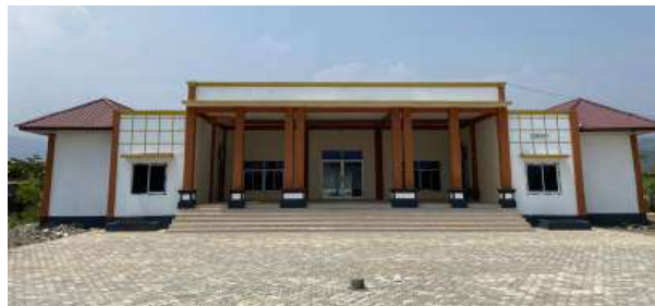
Construction of Le-le Village Office
