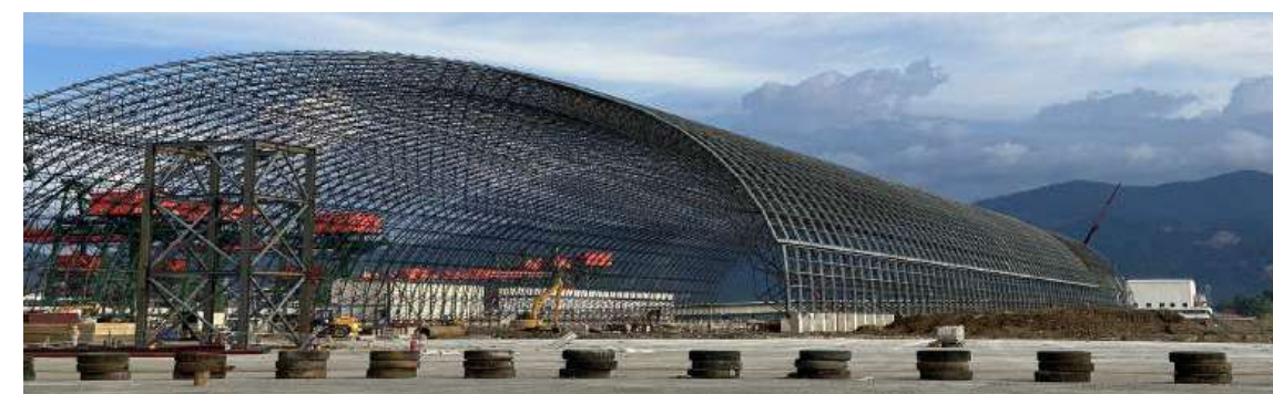
large coal shed
