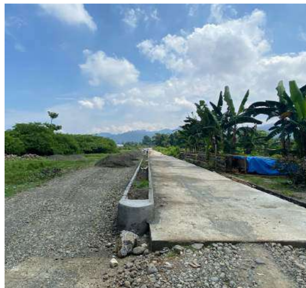
The road pavement project in
