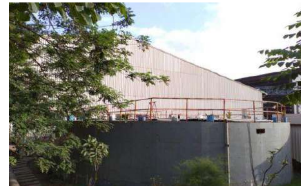
Domestic Sewage Collection Tank
