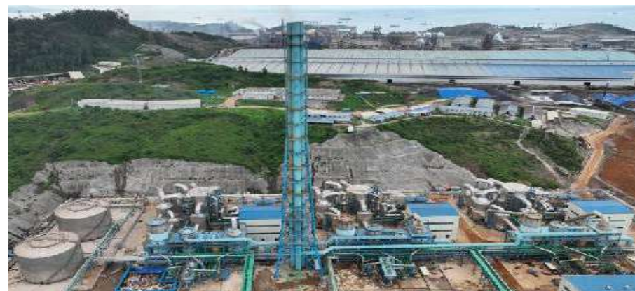
PT.HYNC 2x25 MW Power Plant
