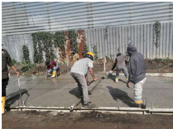
Sulawesi Provincial Road Repair
