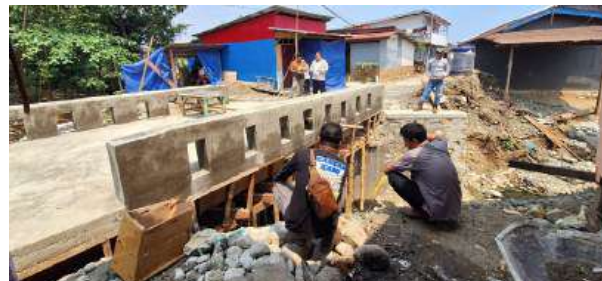
Bridge construction at the second location in District 5 of Bahomakmur Village
