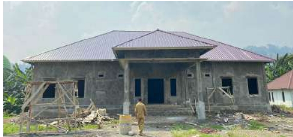
Makarti Jaya Village Office Construction
