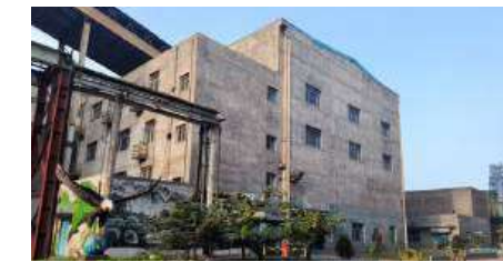
PT.DSI 1*15 MW Waste Heat Power Plant
