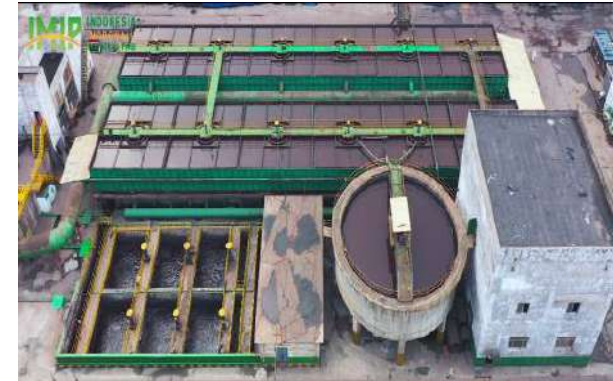
Production Wastewater Treatment Station
