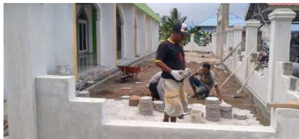
Construction of Annaja Mosque in Bete-Bete Village
