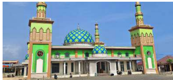
Construction of the minaret of Nurul Taqwa Mosque
