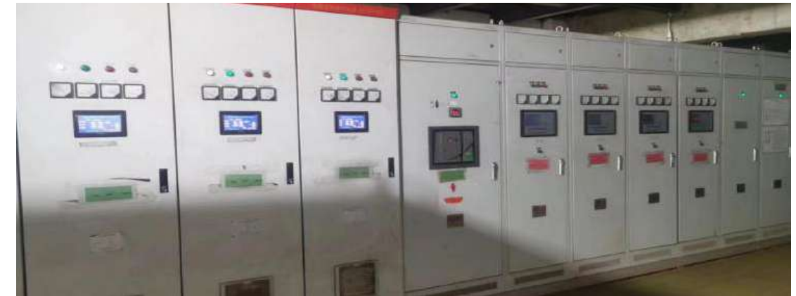
Intelligent Pulse Frequency Conversion Control System for Electrostatic Precipitator
