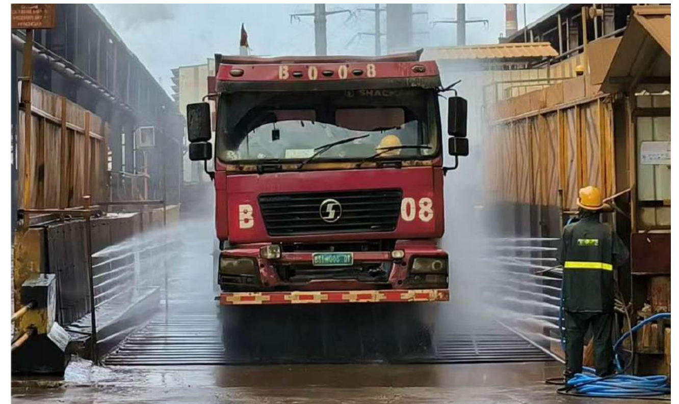
Rainwater is recycled for car washing at the car wash station
