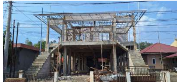
Construction of Lalampu Village Hall
